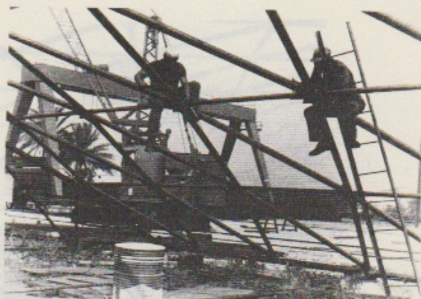
Fig. 17.15. The experimental prototype barrel vault erected for testing in Ondara, Spain.
