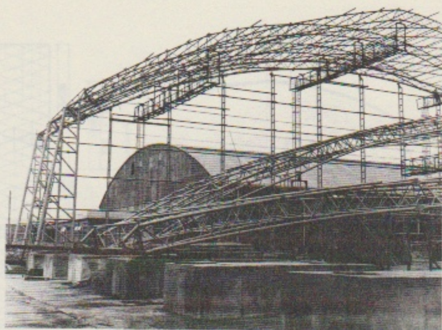
Fig. 17.13. Lamella latticed barrel vault for greater spans (the Berlin ice stadium).
