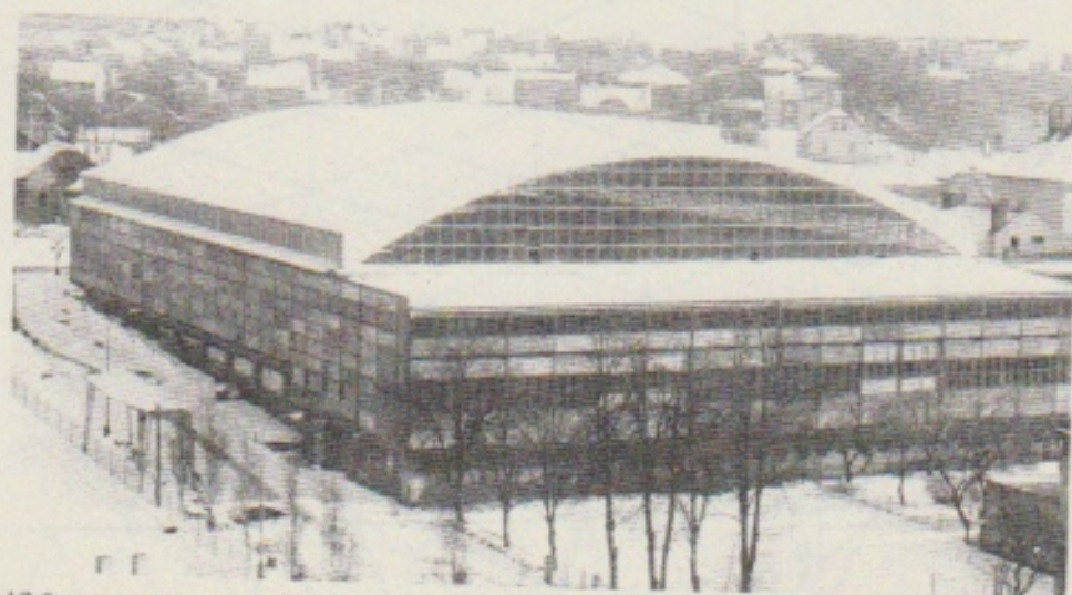
Fig. 17.9. The simple architectural treatment of the lamella barrel vault over the ice rink in Kopřivnice.
