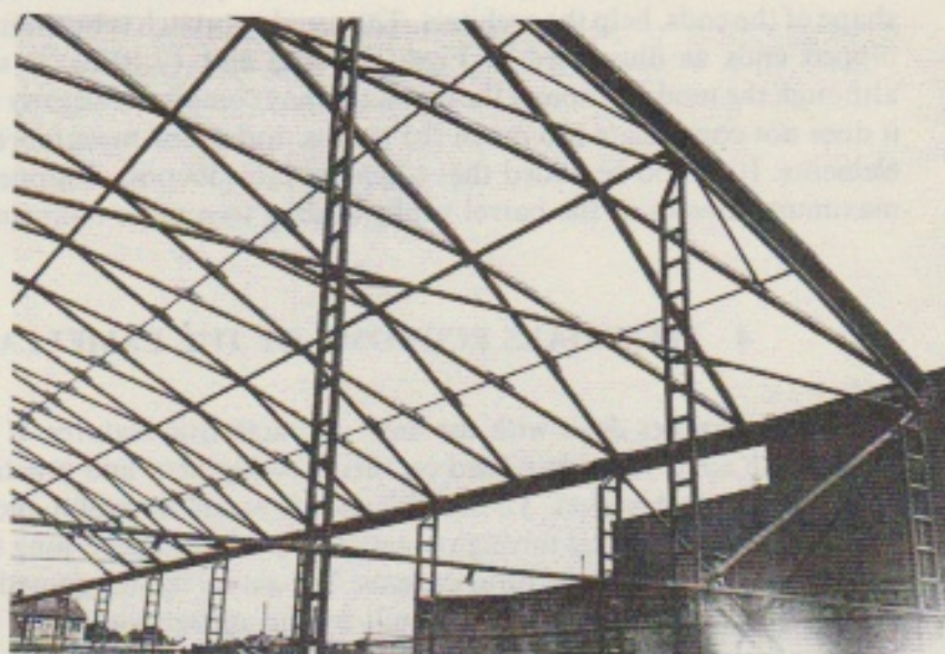
Fig. 17.11. A typical example of a slender single-layer lamella barrel vault.
